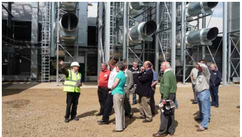
Guests toured the newly extended site at Whiterashes with its new grain drying, office and strage facilities
